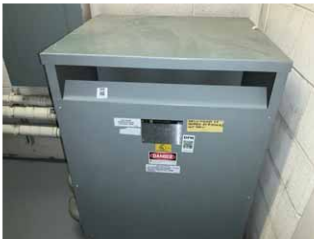
39 - SECONDARY TRANSFORMER
