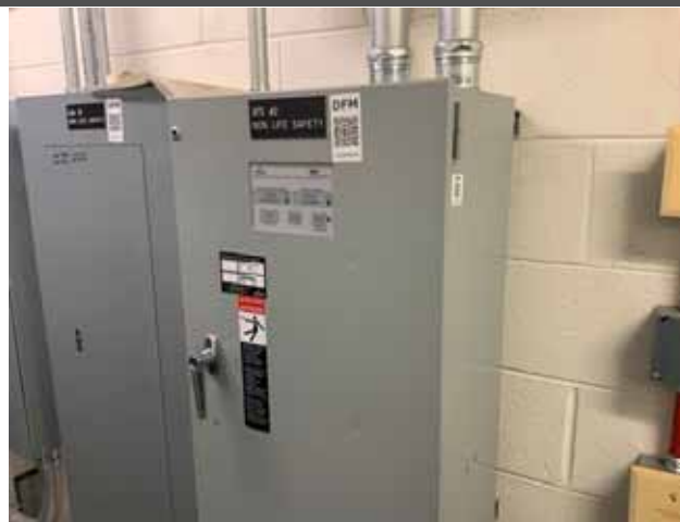
38 - AUTOMATIC TRANSFER SWITCH
